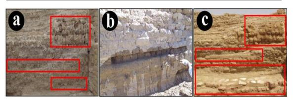
Fig. 14. The method of restoration and filling the missing parts in mud brick buildings (a) Some disintegrated mud brick courses in the wall, need to be removed and rebuilt, (b) During rebuilding with modern mud bricks and mud mortar, (c) The wall after rebuilding.
