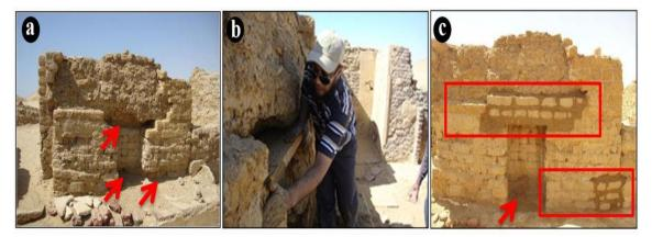
Fig. 15. Steps of the initial restoration of the niche (a) The niche wall before restoration, (b) During restoration and inserting the wooden lintel, (c) The niche wall after initial restoration.
