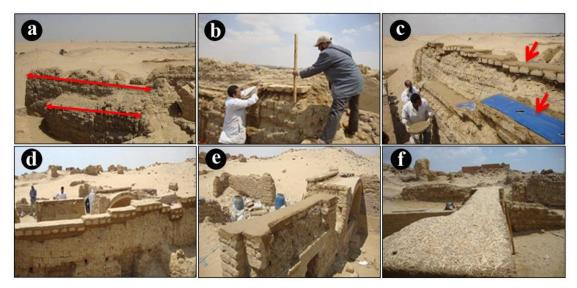
Fig. 16. Steps of reconstruction and capping of upper courses in adobe walls (a) Some adobe walls, the upper courses of which were completely destroyed by rain water and other atmospheric agents, (b, c) During reconstruction and capping using mud bricks, mud mortar and plastic sheets, (d, e, f) Some adobe walls after reconstruction and capping.
