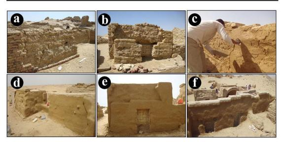
Fig. 17. The technique of troweling with mud plaster (a, b) Some mud brick walls before plastering, (c) During plastering "troweling", (d, e, f) Some mud brick walls after troweling with mud plaster.
