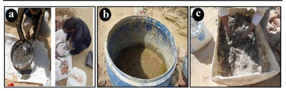
Fig. 10. Stages of preparing the mud mixture for manufacturing mud bricks, and preparing the mortar mixtures used in different restoration works (a) Sieving the ingredients and purify them from impurities, (b) Fermentation process, (c) Kneading process.
