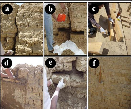
Fig. 13. Mud brick walls before, during and after treating the cracks (a) A cracked wall before treatment, (b) Making a rectangular hole in the wall perpendicular to the crack, (c) Treating the wood beams with the pesticide, (d, e) During reconnecting the cracked wall using wood beams with mud mortar and mud bricks, (f) The cracked wall after treatment.
