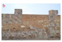
Fig. 14. (a) Collapse of Parts of the Building, (b) Erosion of Mortar Layers and the Building's Limestone
