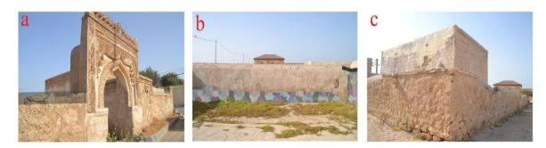
Fig. 18. Deterioration Phenomena in Hussein Al-Rifai's House: (a) where Parts of the Building Collapsed, (b) The Falling of Casing Layers and Mortars, (c) Inappropriate Restoration Work
