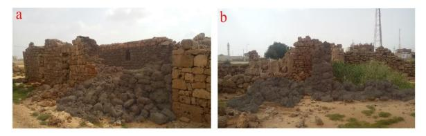
Fig. 8. (a) The Collapse of Large Parts of Al Arady Buildings, (b) The Effect of the Biological Damage
